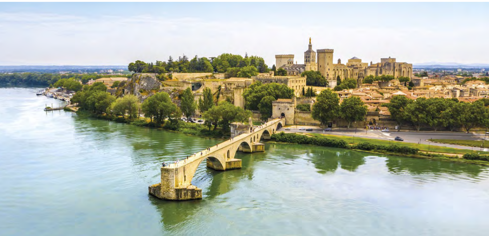
St Benezet Bridge, Avignon, France
