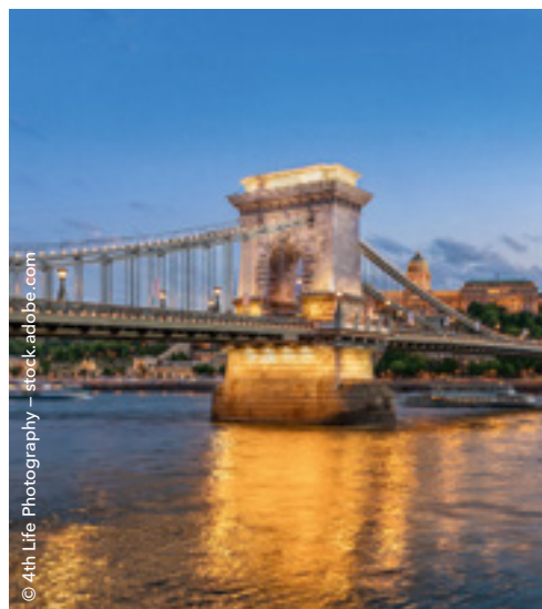
Budapest: Chain Bridge
